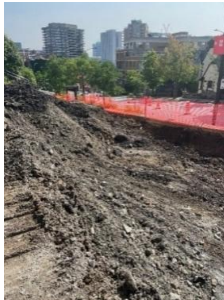
Construction work at the Montreal General Hospital emergency entrance. As part of the installation of stormwater retention basins, 1,335 metric tonnes of A-B quality soil and 592 metric tonnes of B-C quality soil were transported off-site and recorded in Traces Québec.
