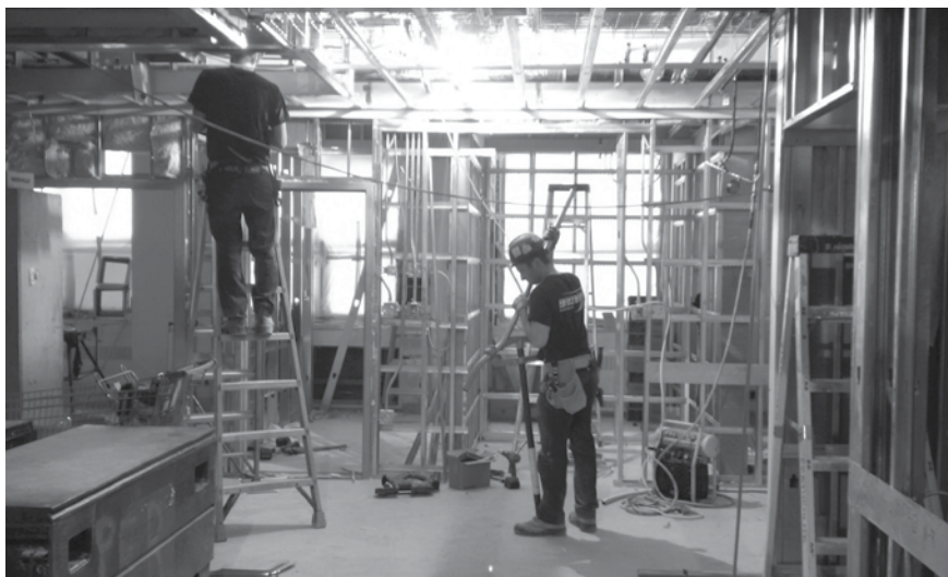
This construction area is destined to become the only psychiatric emergency department for adults at the MUHC, with some 3,000 visits per year expected.
